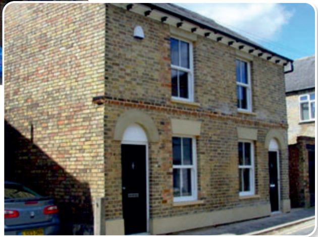
23/24 Great Northern Street, (After)
